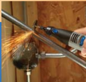
Cutting an iron pipe
