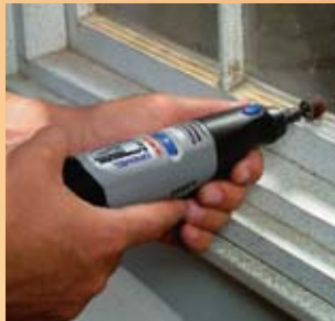
Removing old putty
