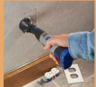
Cutting a hole in a drywall
