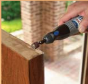
Sanding wood to unstick a door
