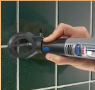
Removing old grout between tiles
